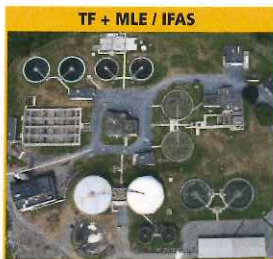
Figure 6: Facility in the Chesapeake Bay Watershed (Facility A).
